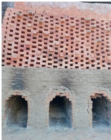
Fig. 4. Burning of brick
