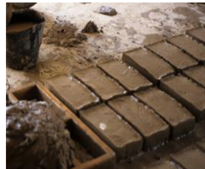
Fig. 4. Brick Moulding Process
